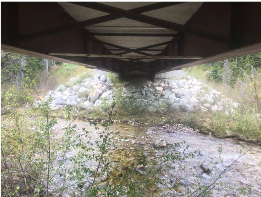
Left Bank Abutment when facing downstream
